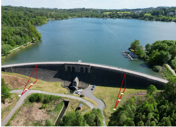
Figure 2. Measurement setup at the Brucher water dam, where two scanning lines were placed on each side at distances of 10 m, 20 m, and 30 m, represented by white points.
