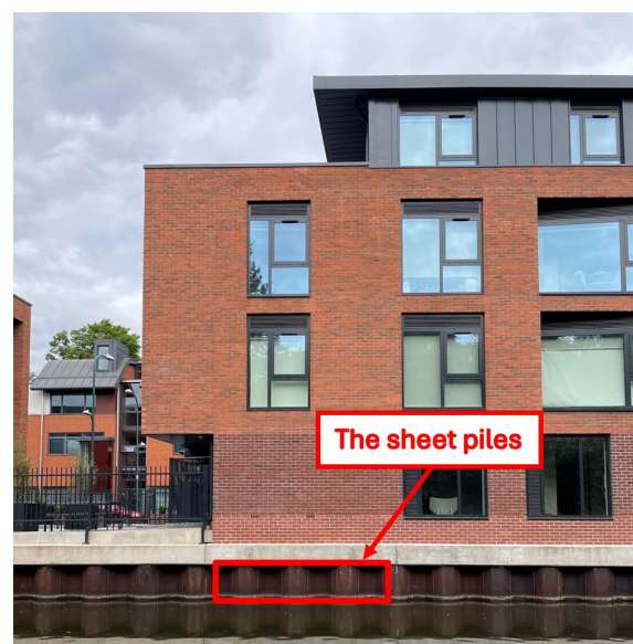
Figure 1. The monitored part of the sheet piles. The red box has dimensions of 3.5 m x 1 m.
