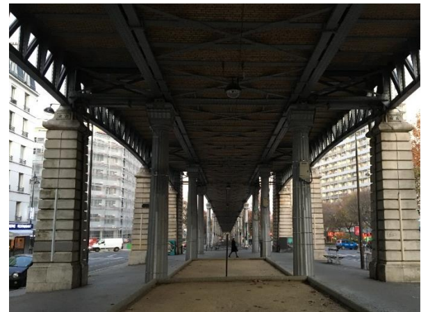
Figure 4. Under the viaduct of the Line 6: vertical OS sensors are set on the masonry piles and protected by half-pipes. EDAS are installed at the top of selected piles.
