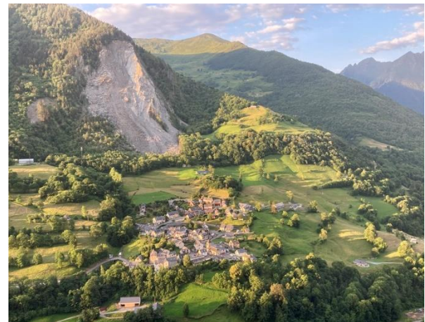
Figure 7. Viella landslide in August 2020 (France)
