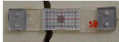
Fig. 6 View of a crack meter installed inside the Mieroszewski Palace
