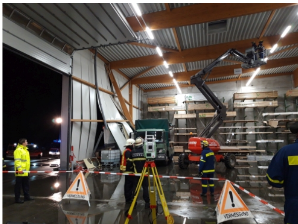
Figure 7. Monitoring of a damaged industrial building after a truck collision, picture: Andreas Knöpfler THW OV Landau
