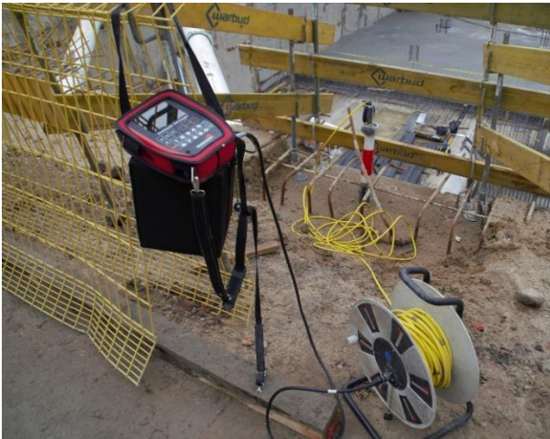
Figure 6. Inclino-metric measuring system at the measuring station
