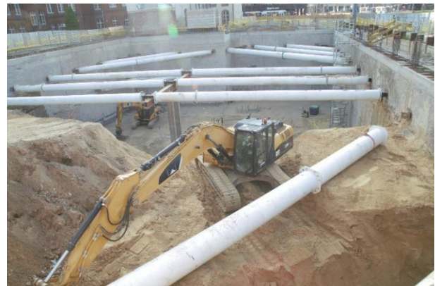
Figure 3. Construction site - diaphragm walls and struts during earthworks
