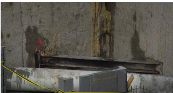
Figure 2. Sealing the joints of wall segments by injection
