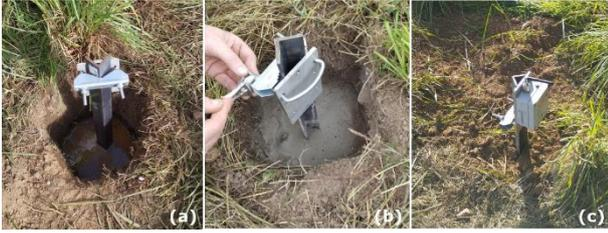
Figure 2. Installation of tiltmeters: (a) a 80 cm angle steel beam is fixed in a 30 cm × 30 cm × 30 cm posthole using postcrete and buried at 50cm depth, (b) a mounting plate is firmly fixed on the angle steel, (c) the tiltmeter is mounted onto the plate. Final position at 20 cm above ground surface.
