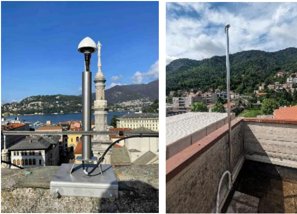
Figure 4. Installations of new GMUs in stations HEM4 (on the left) and HEM5 (on the right).
