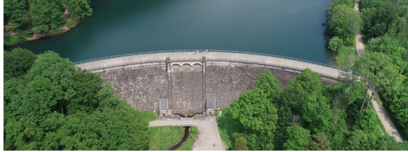
Figure 1. Jubach dam photographed with a drone from the land side.
