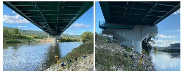
Figure 8. Used interferometric radars: Left - Bottom view on the bridge deck with the steel crossbeams from the position of the radar R1; Right - View on both radars: R1 is in the foreground, and R2 is in the background in the photo.
